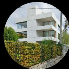
apartment building Prule, Ljubljana
