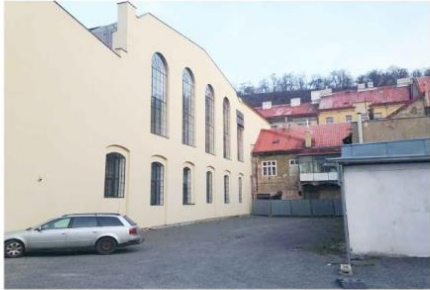
ECONOMIA FACADE - PART OF THE FUTURE COURTYARD
