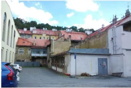
BACK ADDITIONS TO EXISTING BUILDINGS - DEMOLITION
